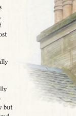
with cement where the stone has decayed. The junction between chimney stalk and roof is a weak point in the roof covering and any deterioration of the lead flashings or cement fillets here should be repaired promptly.
